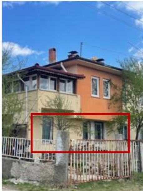
Figure 11. Conversion of stable-designed ground floor into residential space (Baran Ergül, 2025)
