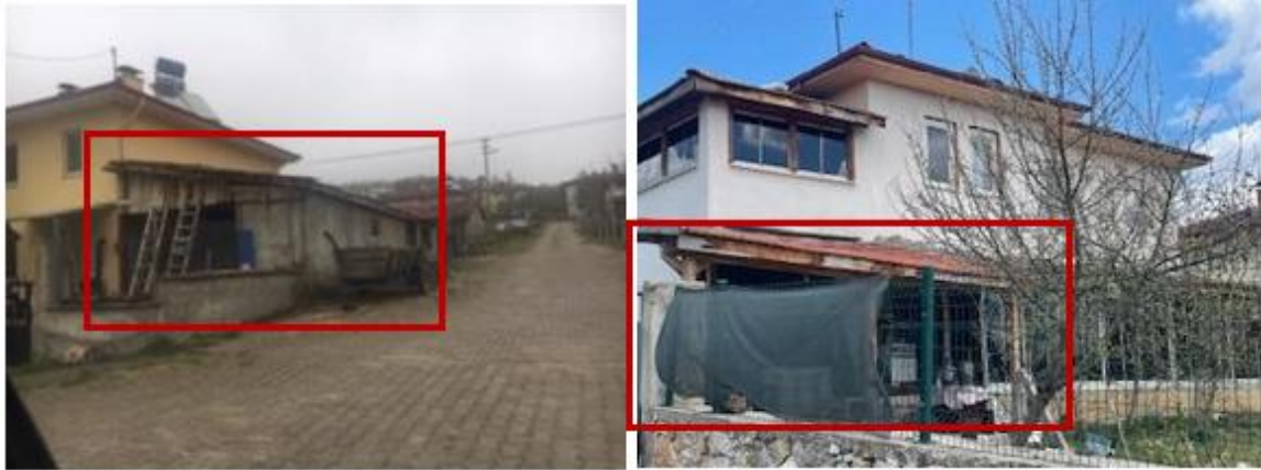
Figure 8. Ancillary structures adjoining the dwelling: animal shelters and garages (Baran Ergül, 2025)
