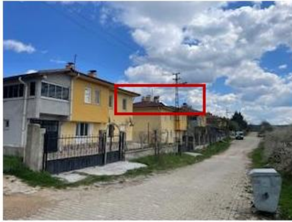
Figure 10. Installation of solar thermal collectors on roofs (Baran Ergül, 2025)
